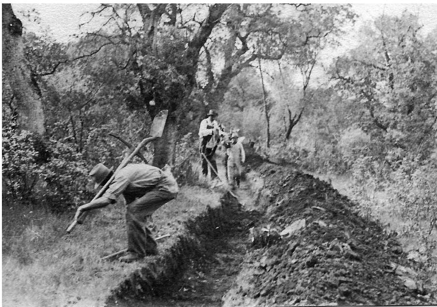
Workers construct the Reille Ditch in Placer County during the 1930s
