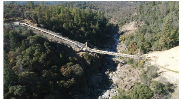
The aerial siphon crosses the Bear River.
