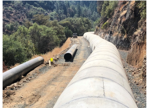
The Combie Phase 1 pipeline stretches 1.7 miles.
