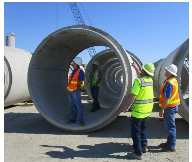
Inspectors look over the massive pipe segments.
