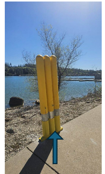
Recreation staff built these receptacles for the bollards; it allows safe storage during launching hours.
