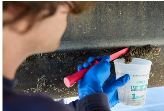
A worker scrapes Golden Mussels from a pontoon on a work barge at a Delta boatyard. Photo CalMatters
