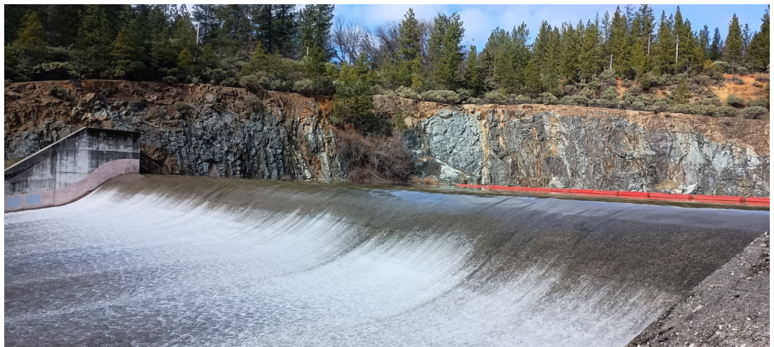
Rollins Dam spills on Feb. 18, 2025
