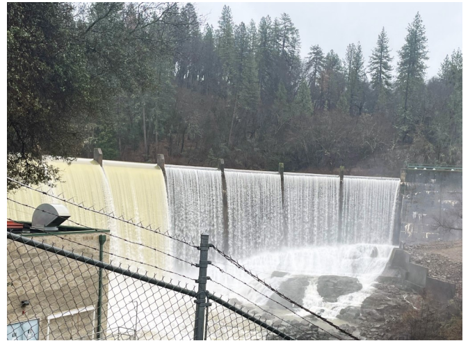
Van Giesen Dam (Combie Reservoir spills on Feb. 6, 2025)
