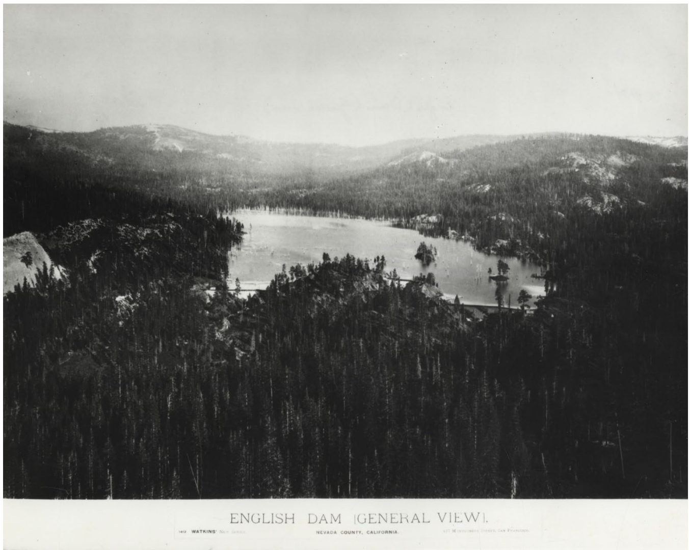
Figure 3. Overview of English Dam, c. 1871 (Source: California State University, Chico, Meriam Library Special Collections).
