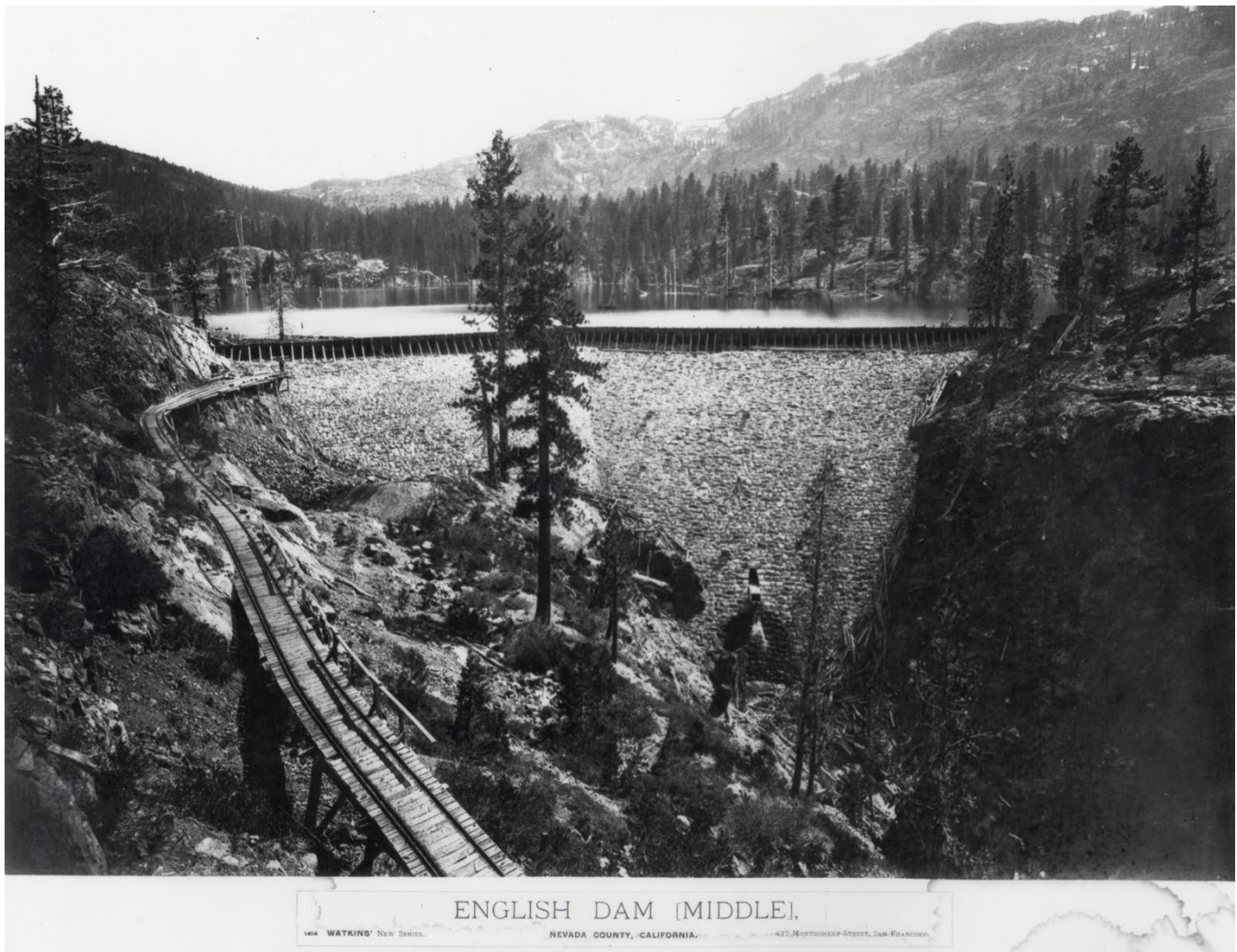
Figure 6. Overview of main dam, c. 1871 (Source: California State University, Chico, Meriam Library Special Collections).
