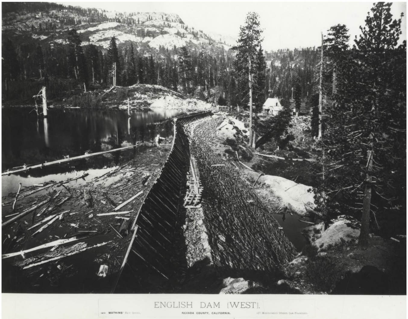
Figure 5. Overview of west saddle dam, c. 1871 (Source: California State University, Chico, Meriam Library Special Collections).
