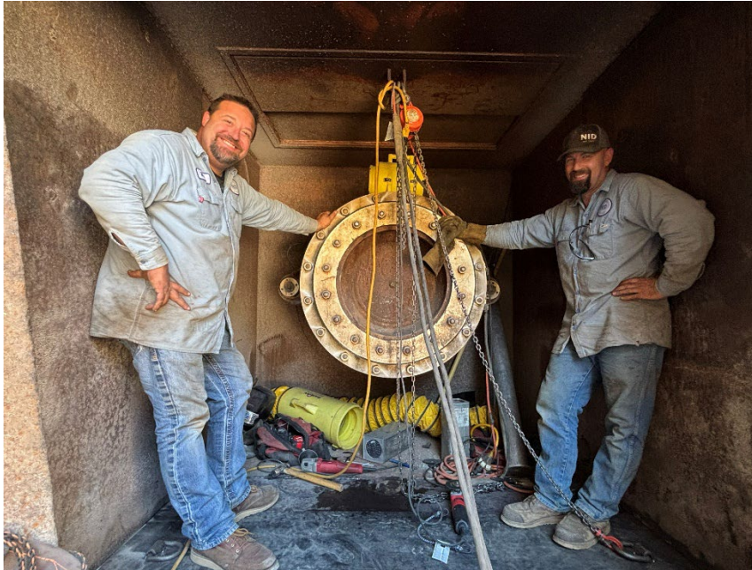
Senior Welder Robert Stice and Welder II Josh Pratt work on the PRV.
