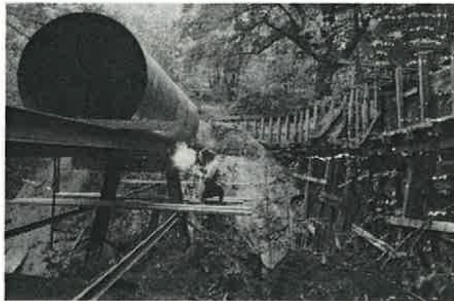
STEEL PIPE is replacing an old wooden flume in the current project on the Cascade Canal. The five-foot pipe is being supported on 10-inch I-beams.
