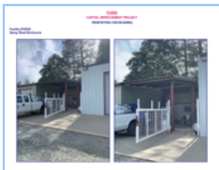
Spray Shed Enclosure
