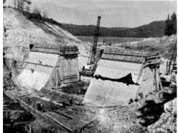
Building Scotts Flat Dam, 1964
