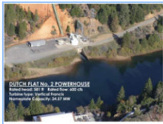
Dutch Flat #2 Powerhouse
