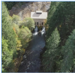
Deer Creek Powerhouse
