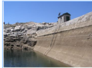
French Dam Gate House
