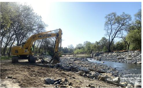
The dam, which was a barrier to fish, is being replaced with a system that opens up approximately six miles of habitat to migrating and resident fish on the upstream side of the diversion. The new system also allows water delivery to customers via the Hemphill Canal. First flows occurred in November 2022.
