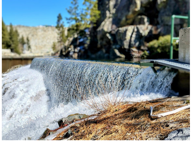
Overflow between Bowman afterbay before it enters the Bowman canal (March 12).
