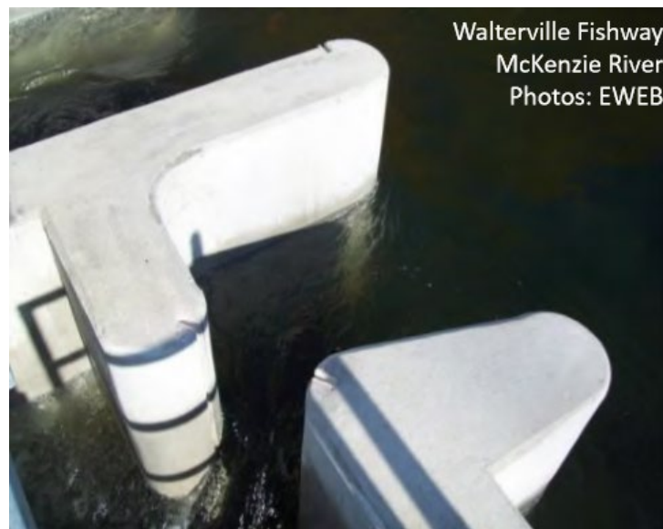
Figure 3-5. An example of a vertical slot fishway with rounded corners for Pacific Lamprey passage. Lamprey passage is improved in fishways when concrete corners are rounded with a 3-4 inch radius. Photo credit: Eugene Water and Electric Board
