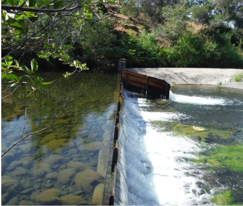
Figure 3-7. Example of a removable fishway structure on a diversion dam installed during diversion season (while flashboards are currently installed). Photo credit: NHC
