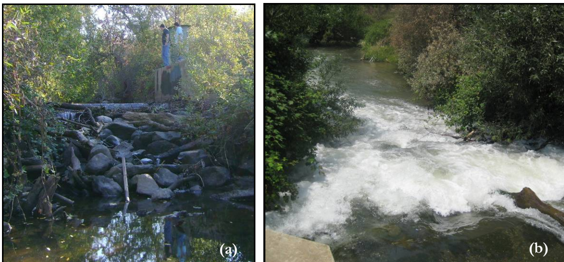
Figure 1. A riprap ramp leading up to the NID flow gaging station, which consists of a 25-foot wide concrete Parshall flume. At low flows (a) water depths are too shallow for fish passage. At higher flows (b) water velocities and turbulence can become excessive for passage of adult and juvenile salmonids.
