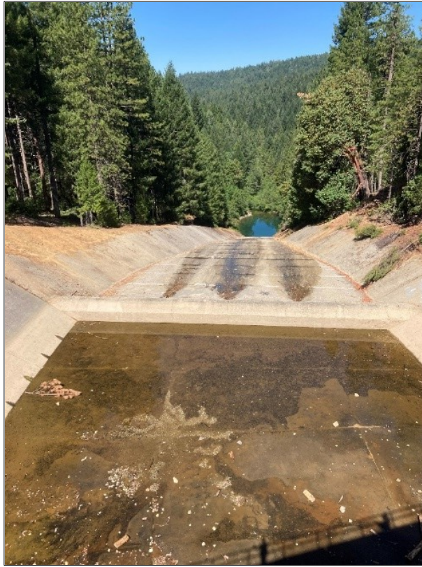
Photo 2-11: Upper Plunge Pool and Upper Spillway Chute
