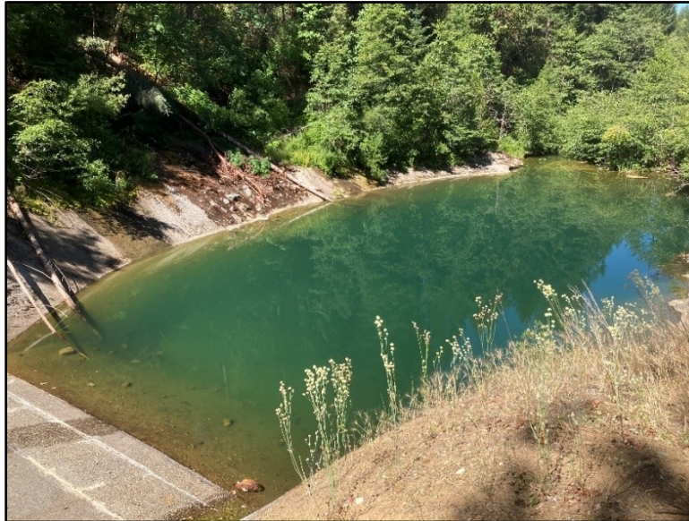
Photo 2-2: Existing Lower Plunge Pool
