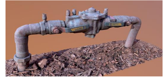
Reduced Pressure Prevention Assembly (RP)
