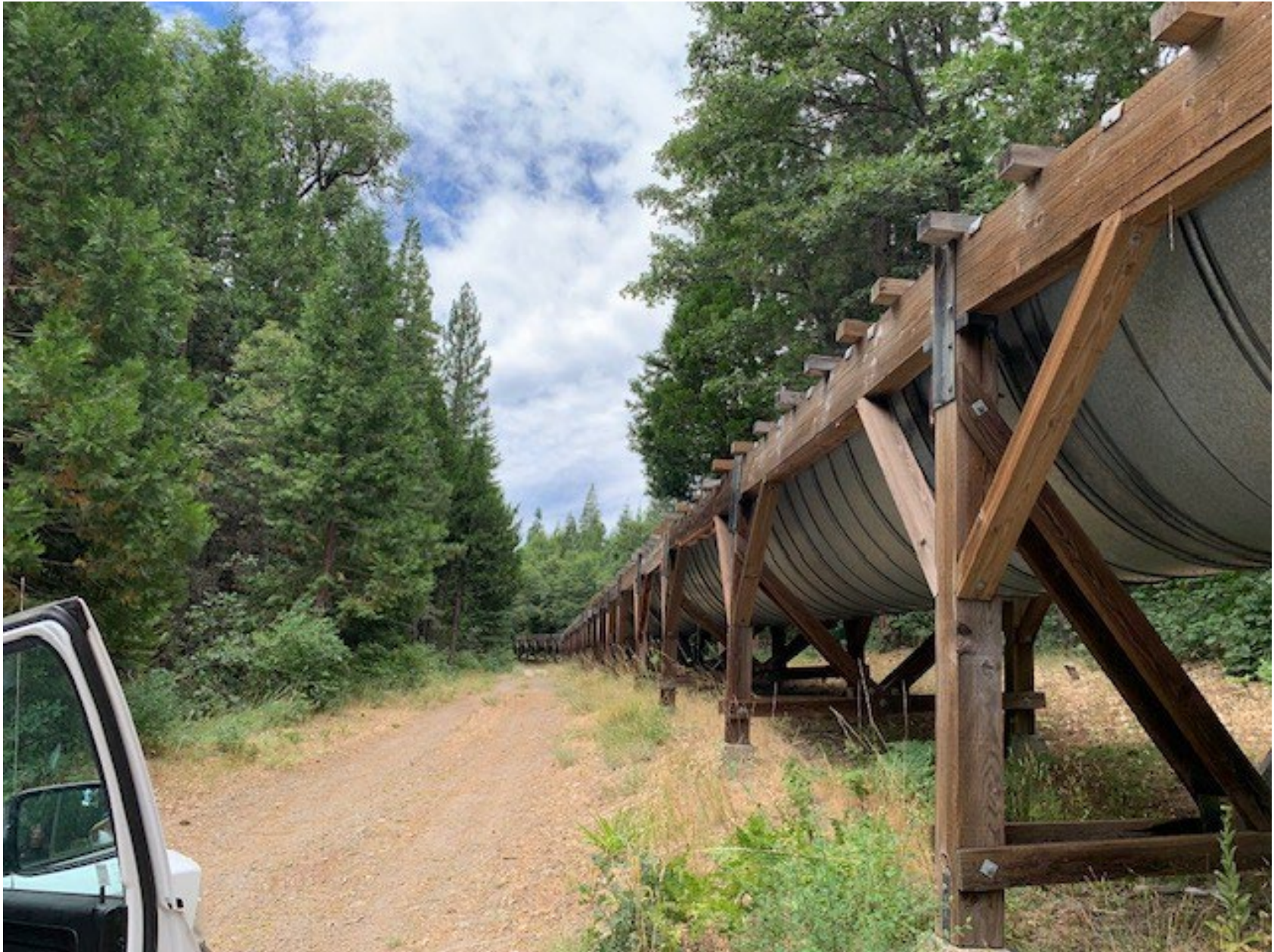
South Yuba Canal with access road downhill of raised flume
