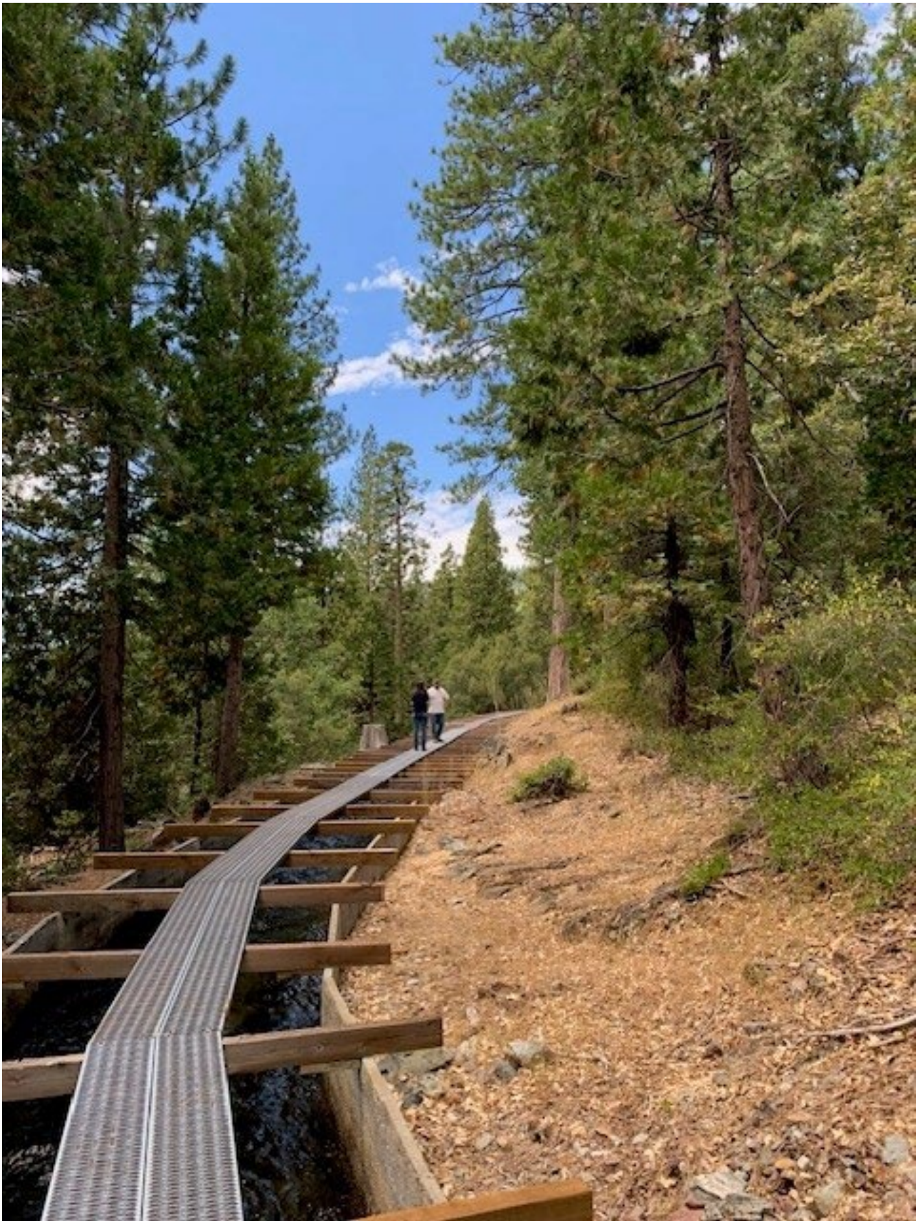
South Yuba Canal with adjacent vegetation
