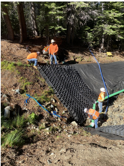
The geogrid is positioned on the slope
