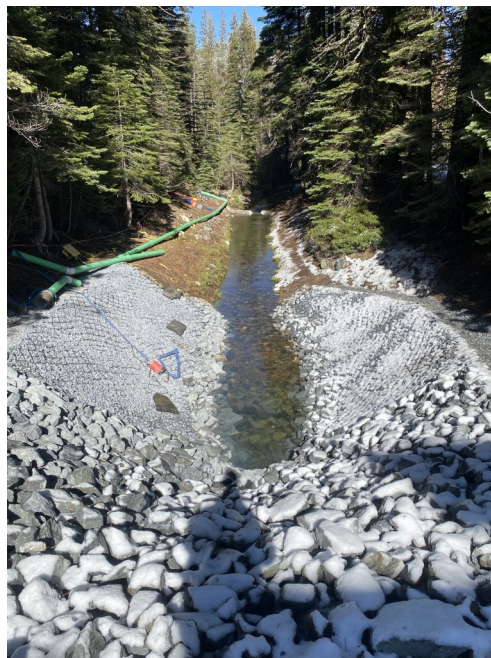
The gravel will stabilize the slopes
