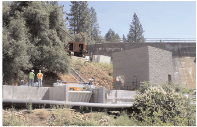
The new 500-kilowatt Combie North power plant is nearing completion.
