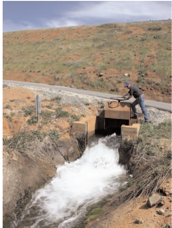
NID Water Supt. Warren Hart releases irrigation water from Loma Rica Reservoir into the Chicago Park Canal.
