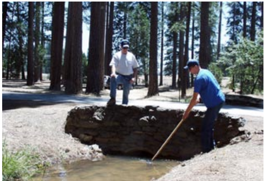
Bill Winkle and Cory Chapman check a culvert on the Allison Ranch Canal at the Nevada County Fairgrounds. NID will have a booth at this year's county fair, Aug. 11-15.
