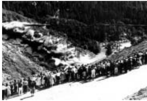
GROUNDBREAKING: A crowd gathered in 1963 when an old Nevada Co. Narrow Gauge Railroad trestle was removed to make way for Rollins Reservoir.
