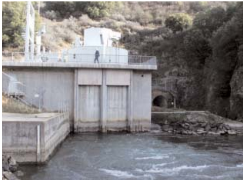
NID's Rollins Powerhouse, in operation since 1980, was the first U.S. power plant added to an existing dam following the 1974 Arab Oil Embargo. NID operates seven hydroelectric power plants.
