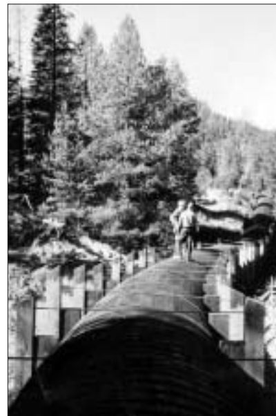
Yesterday Redwood pipe was used in the 1920s for construction of the Milton-Bowman Conduit.
