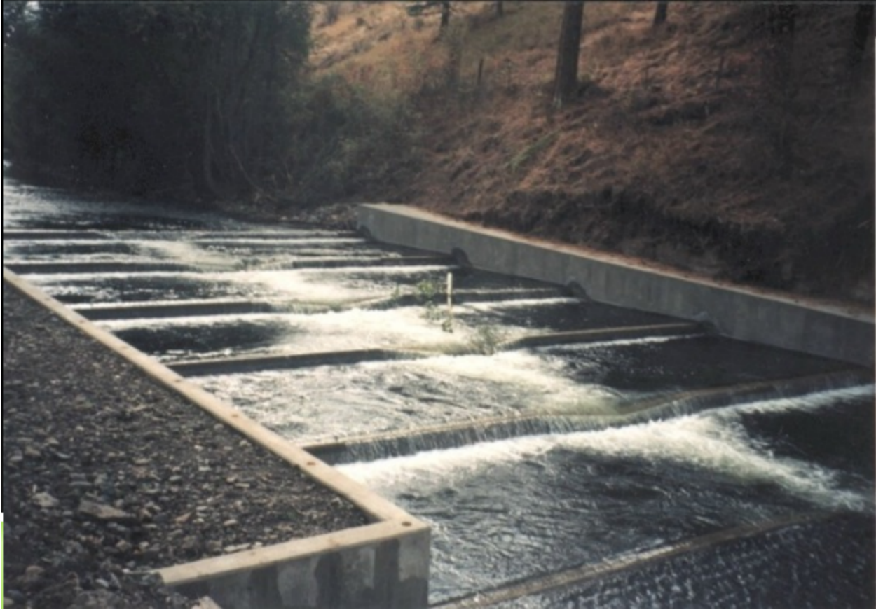
Figure 3-5. Concrete Weir (Pool and Chute) Fishway
