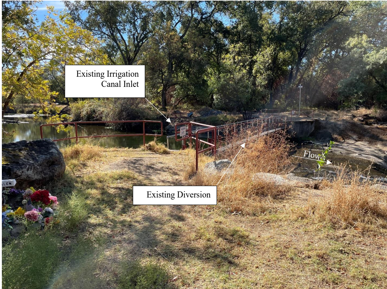
Figure 1-2. Existing Diversion and Irrigation Canal
